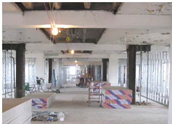
Construction underway at new ADAMHS Board offices in 2010.
