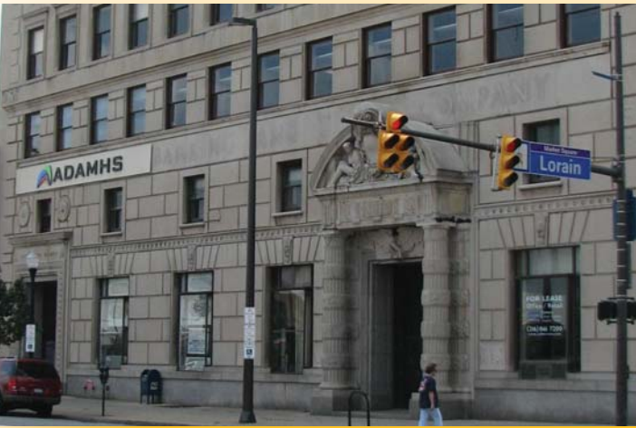
The ADAMHS Board exterior sign was installed on the W. 25 th side of the United Bank building in July 2010. Some people have been referring to the building as the ADAMHS Building.
